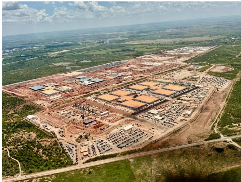
Crédit OpenAI, datacenter Stargate I, Abilene, Texas
